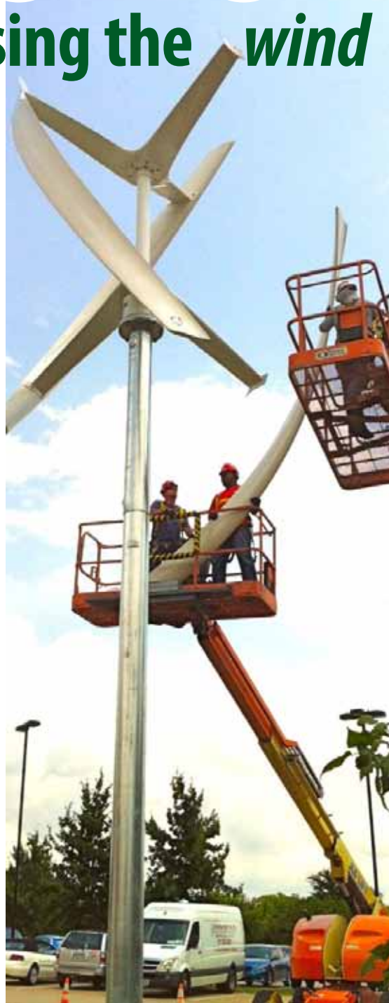
Technicians install the last of three blades on the wind turbine located on the southwest lawn of the Government Center.
